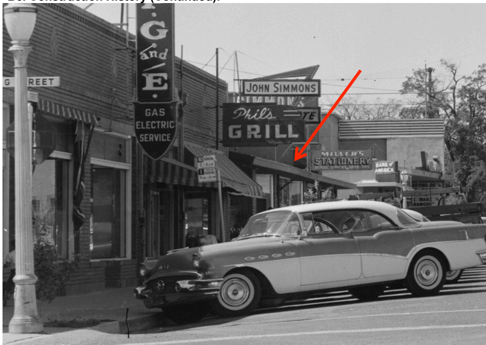
Figure 2. 1960 Photograph of buildings along the south side G Street, taken from 2nd Street looking west. Red arrow points to subject building. (UC Davis Special Collections, Eastman Collection. Amended by author)
